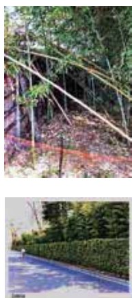
洪水の水勢を弱める竹の生け垣（桂垣） Example for Flood Mitigation; Katsura-gaki flood barrier made of live bamboo can weaken flood energy and let water go through for this barrier structure to withstand.
